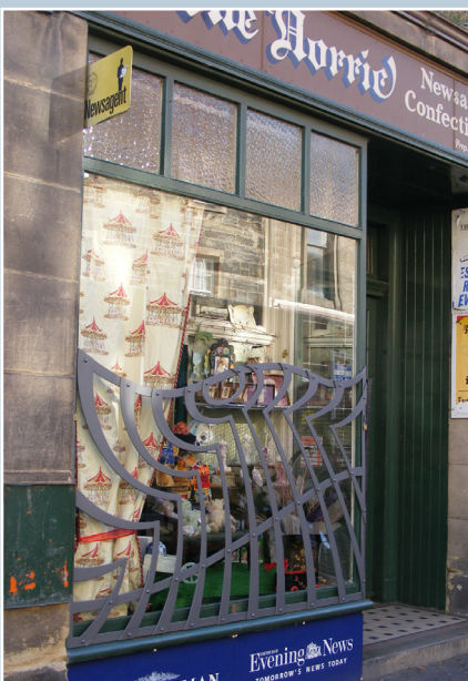
These modern removable external grilles by an artistic blacksmith were put into shops in place of less attractive fixed mesh as part of the Bo'ness Townscape Heritage Initiative.
